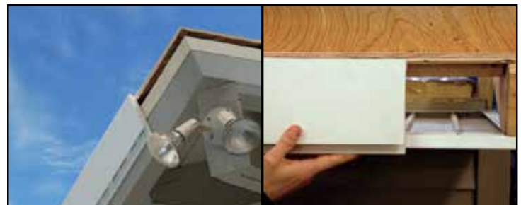
Vented Roof Deck Assemblies
